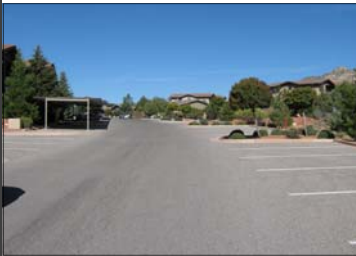
View of installed parking lot.
