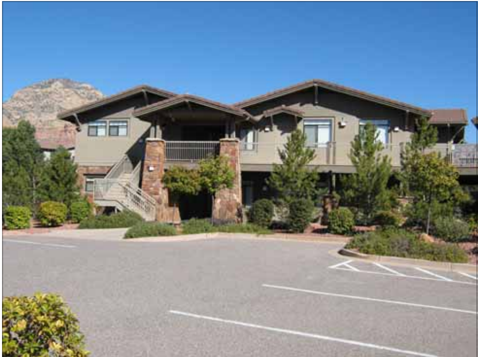
View of completed 12-Plex Apartment Building
