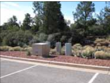
View of installed utilities.
