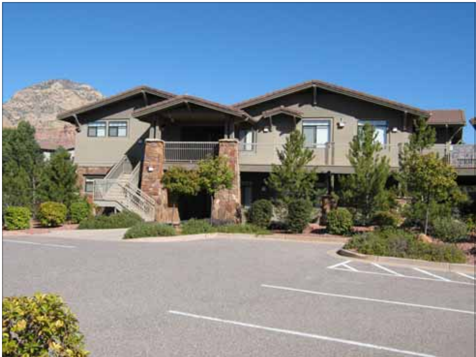
View of completed 12-Plex Apartment Building
