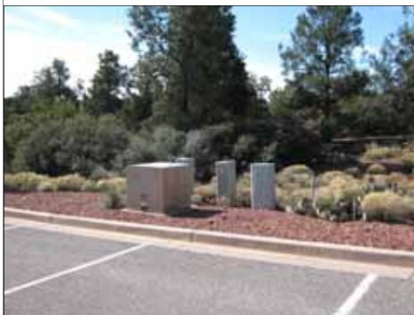
View of installed utilities.
